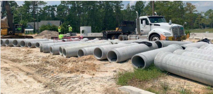
On-site inspection and materials testing at Rivers Edge III
